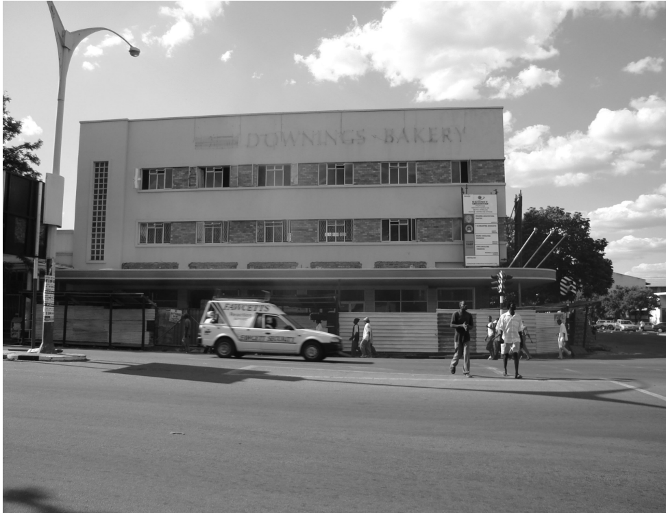
Figure 4.3 Repair and alterations April 2006; formerly Downings Bakery building to be Bulawayo HQ for the mobile phone company ECONET Pvt (Ltd). Corner of Robert Mugabe and Leopold Takawira Avenue (facing north east). Photograph courtesy of B Mbiba.
